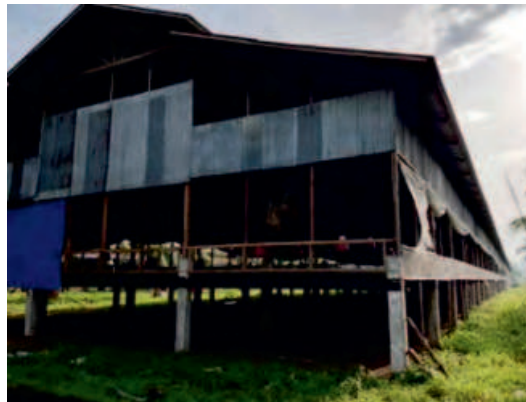
Figure 9.6. High Rised Poultry House.
