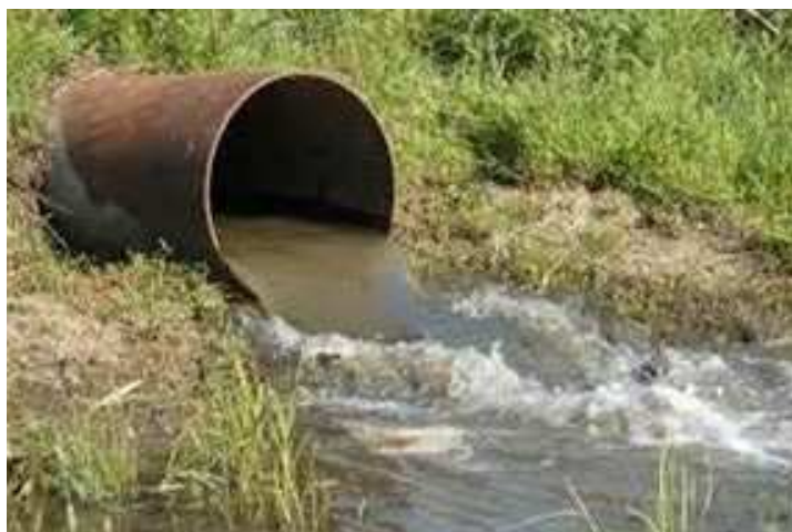
Figure 7.1 Water pollution caused by industrial waste
