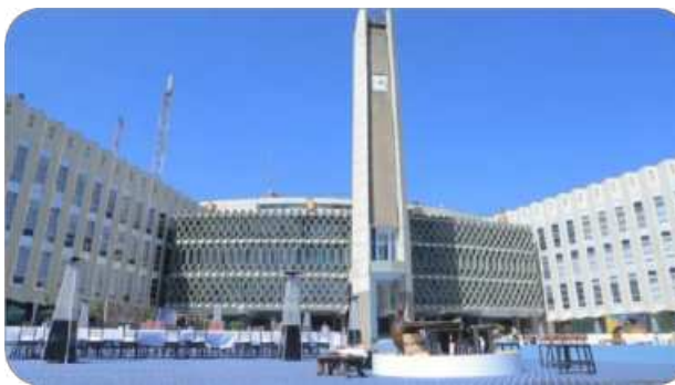
Figure 1.33 Addis Ababa City Hall
